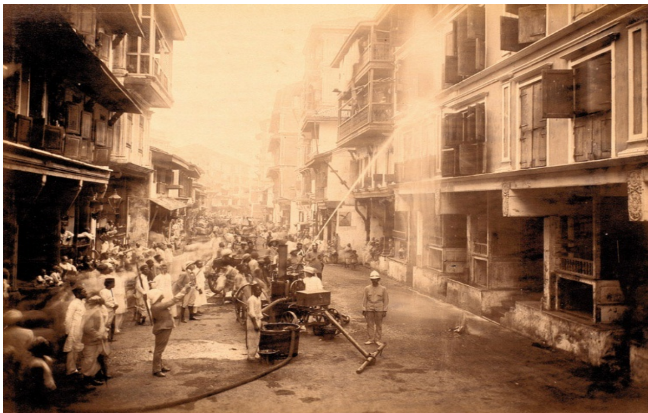
Fig. 9. Disinfection of a House through Flushing Engine, Bombay 1897. 209
